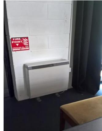
10. Wall hung electric radiator in theater has no guard and is very close to hung curtains
